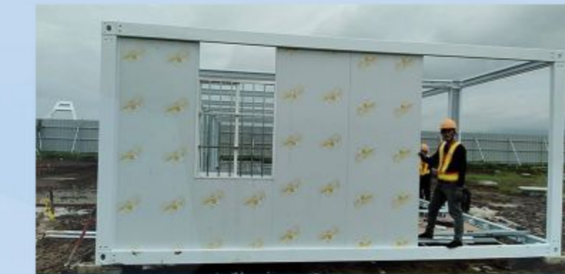
2 . Install wall panels
