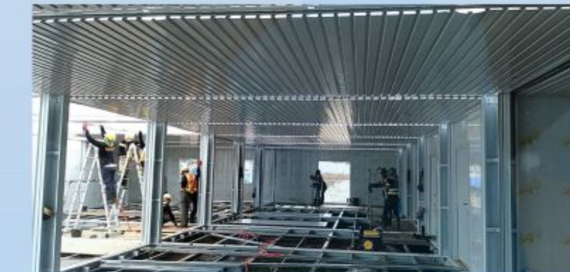
3 . Install windows and doors
